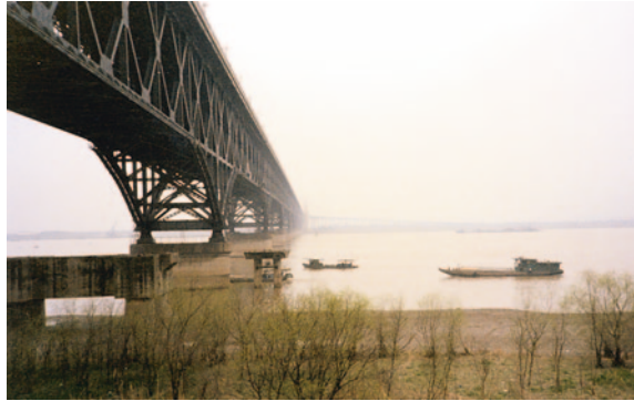
Fig. 6.5 The bridge on the Yangtze in Nanjing, with piers made by the Russians, left unused after political disputes with China
